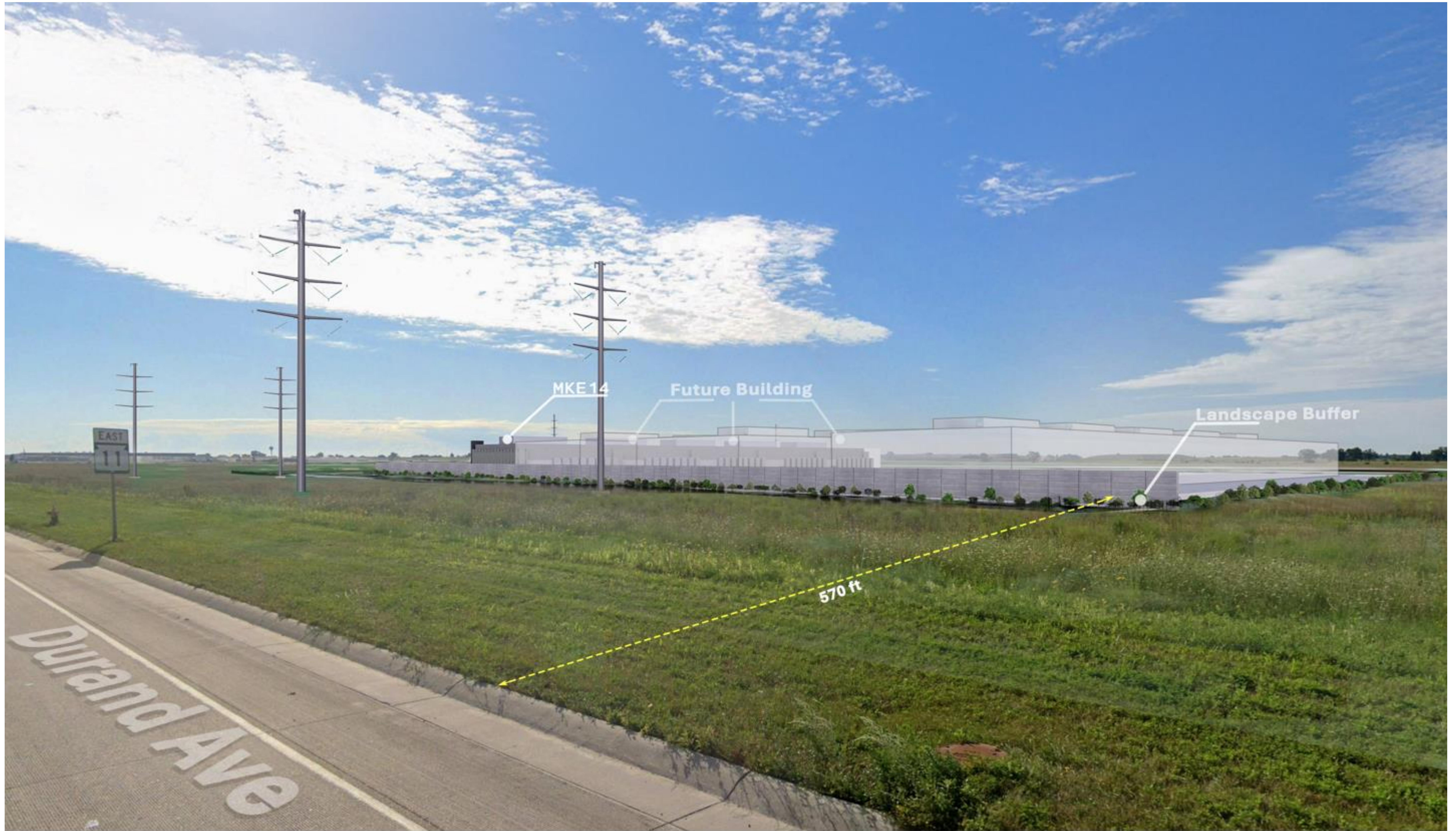
North West View - Durand Avenue
