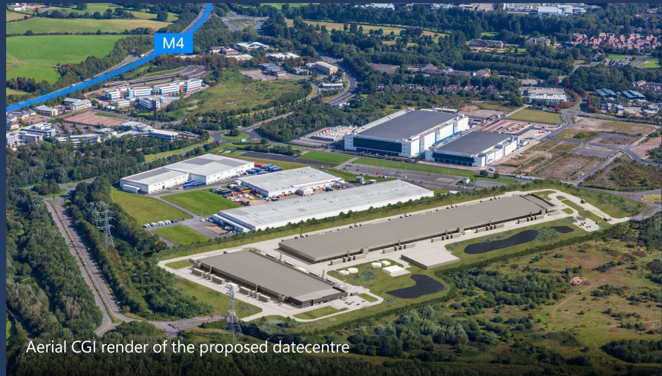
Aerial view of the current site
