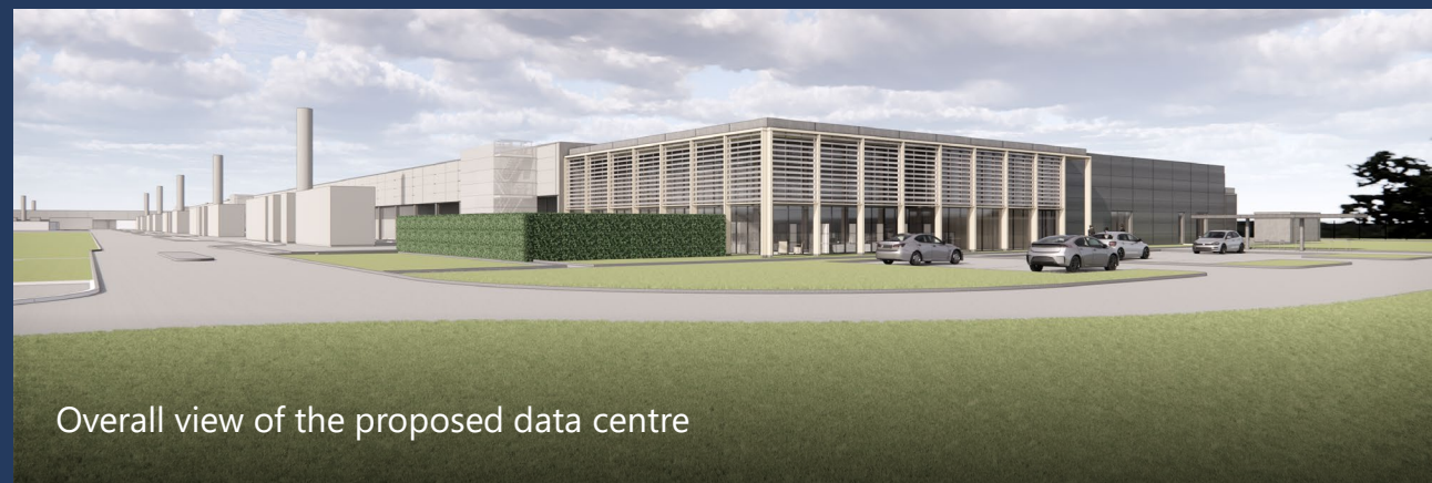
View from the southeast
